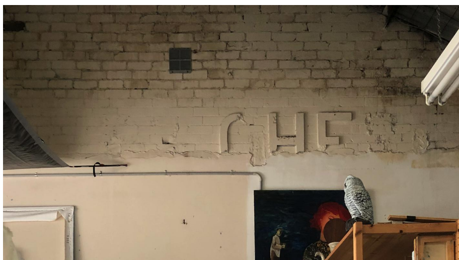
EXISTING "PILCHER" SIGNAGE TO BE RESTORED
