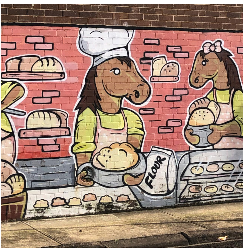
EXISTING MURAL CAN BE RESTORED OR REMOVED
