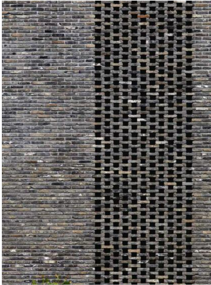
MASONRY SCREEN MAS1
